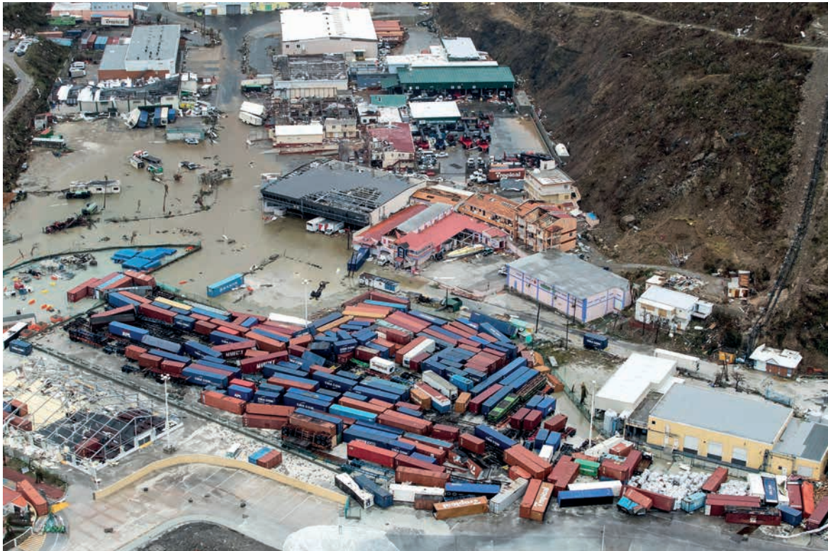
Photo: Overturned shipping containers in Sint Maarten
