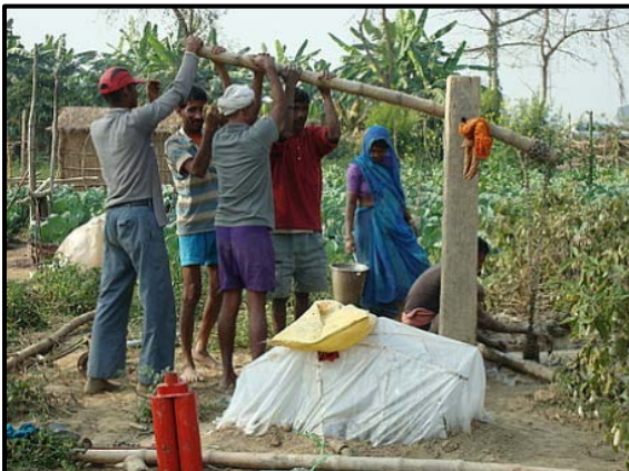
Farmers installing a new treadle pump
