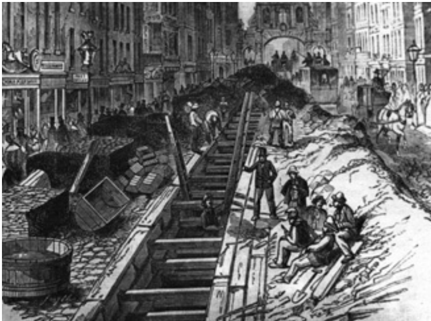
The construction of sewers in London, 1844.
