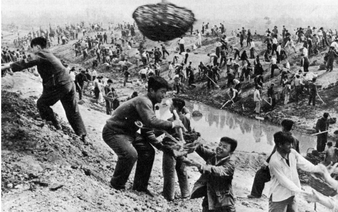
Building a new canal near Beijing during the Great Leap Forward.
