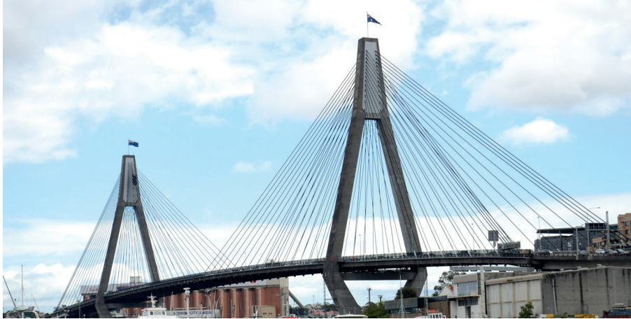
Figure 6: The Anzac Bridge
