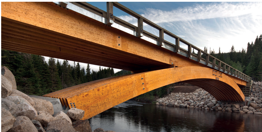
Figure 7: A timber bridge
