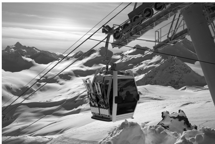
metal wire to support the cable car
